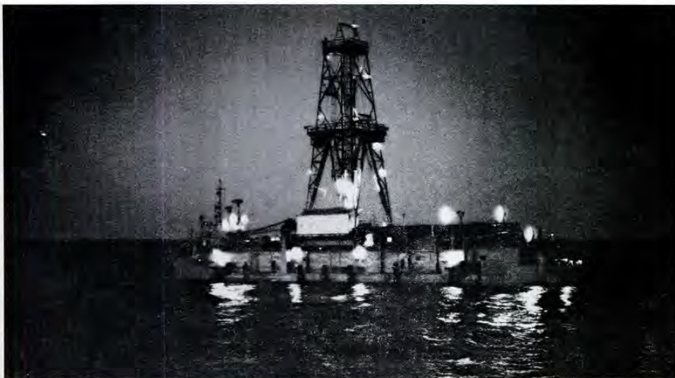
← WORKING THROUGH NIGHT, drillers adjust "kelly" which fits over drill pipe so it can be rotated. Man on high perch (top, center) affixes gauge to measure strain on pipe.
